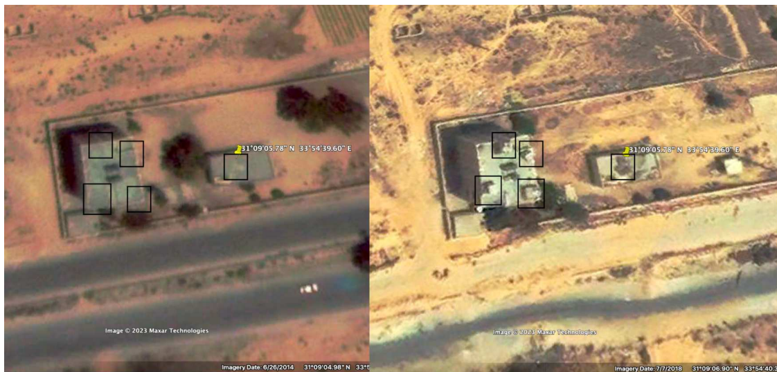
Image 48: The black squares indicate the modern watchtowers built on top of the school's roof. The picture on the right is dated July 7, 2018, and the picture on the left is old before the construction of the towers on June 26, 2014.
