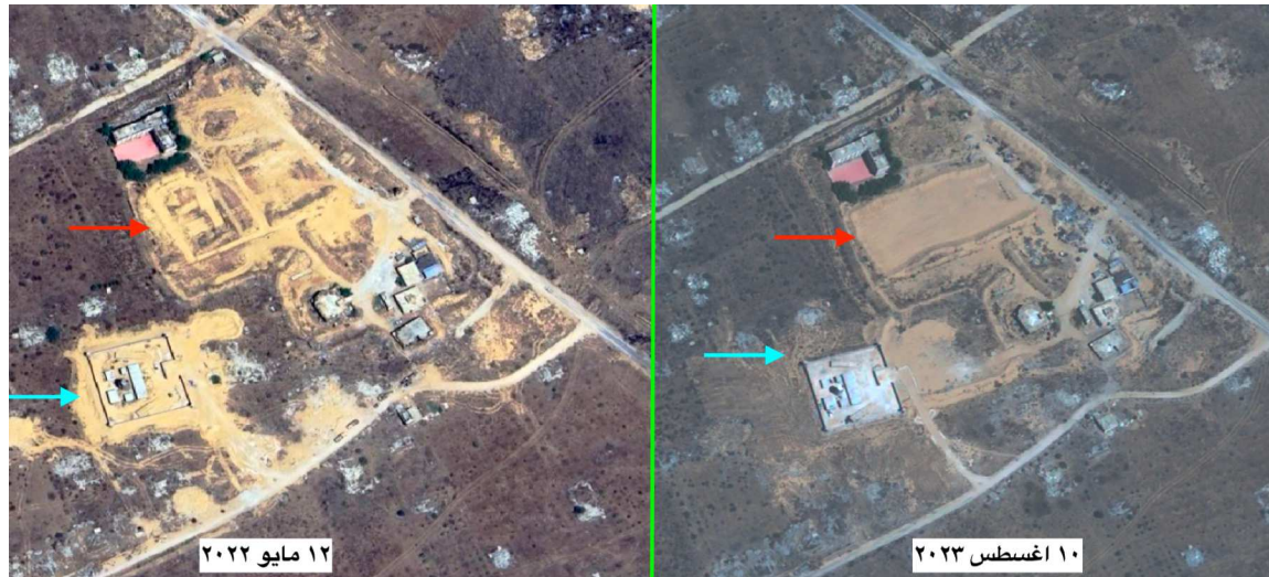
Image 45: The recent image (on the right) shows the continuation of ground paving operations, which indicates the continuation of construction operations.
